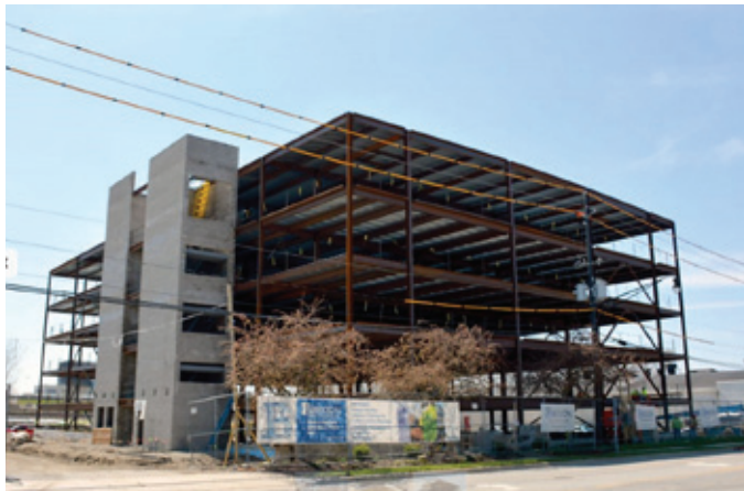
Construction of Tri-Village Self Storage and Brexton headquarters building.
